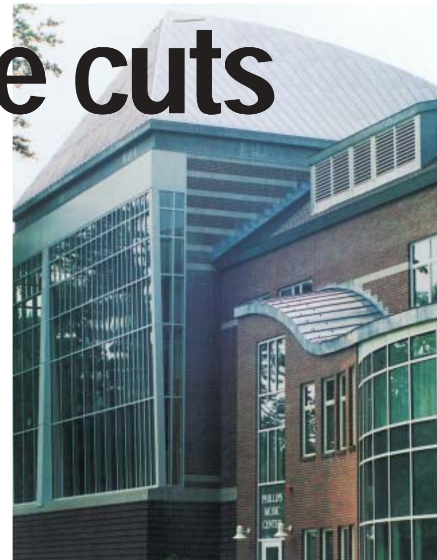
Metal roofing blends in perfect harmony with the brick and glass facade of the Phillips Music Center.
