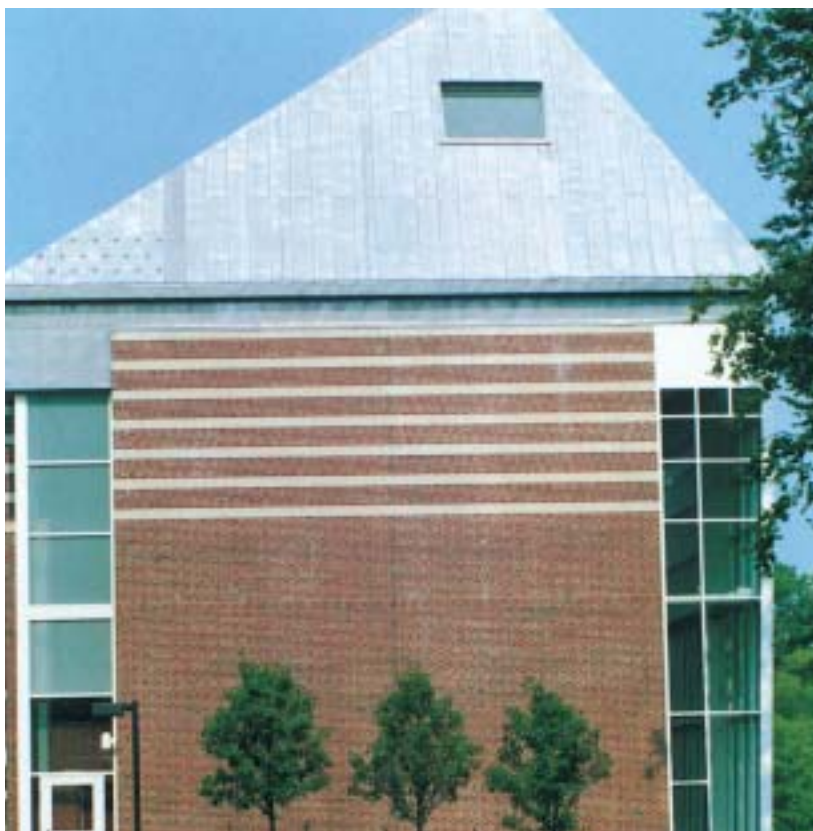
This college building's steeply sloped lead-coated copper roof posed the kinds of challenges relished by A & M Roofing and Sheet Metal, a repeat winner in RSI's metal roofing contest.
